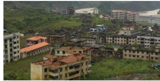
Figure11. Case 2. Collapse of building groups in the south of the town.
