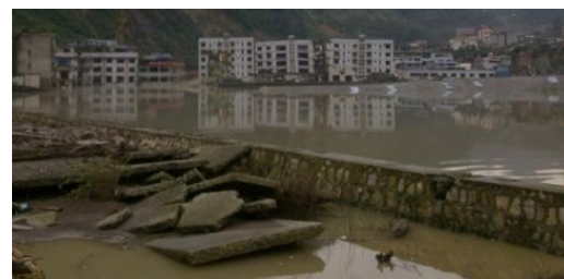
Figure17. Case 7. Landslide near the bend of the Jianjiang in the town.
