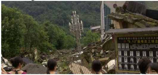
Figure10. Case 1. Collapsed buildings. Before the earthquake this was the Agriculture Bank of China, Beichuan Sub-branch.
