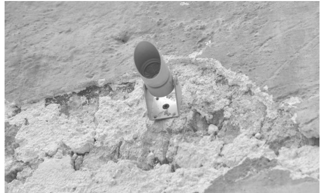
Figure 7. One of the reflectors installed on the Structure's surface.
